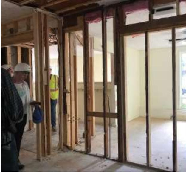
The wall between the coat racks and the sunroom is being removed to create the new lobby.
