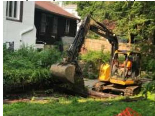
In the back yard, the hazardous materials abatement crew removed asbestos shingles from the north side of the building during the week of July 12. Soon after abatement was completed, a work crew began demolishing the earth berms along the north wall of the building. This work will make way for the addition that will house our new classrooms, hospitality spaces and elevator.
