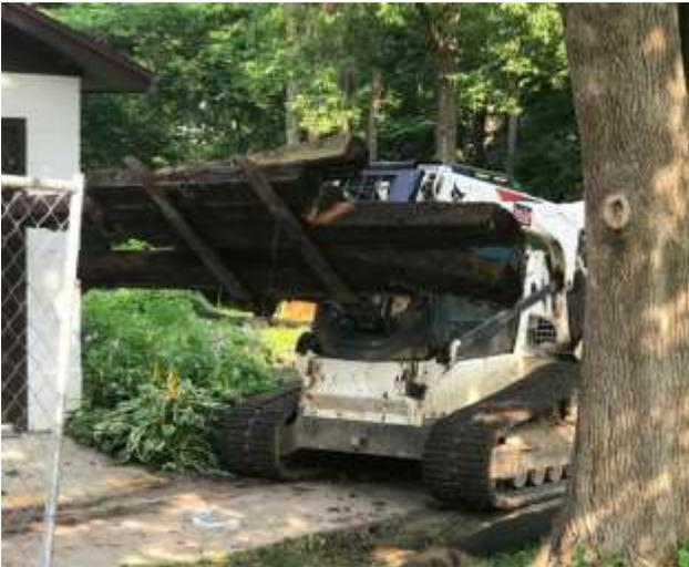
By using small equipment like this fork lift and running it on the sidewalk, Ideal has taken significant steps to protect the maple tree on the northeast corner of the building. Most important, instead of running a large, heavy cement truck into the back yard, they plan to pump cement over the roof of the Meetinghouse.
