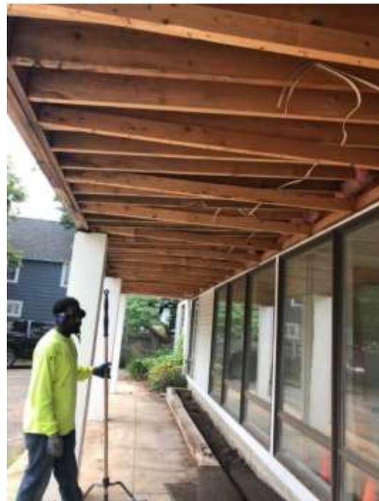
The old portico ceiling was removed due to water damage and discoloration from roof leaks. Fortunately, most of the superstructure was found to be sound. Only a few outer timbers near the post showed signs of water damage and will have to be replaced.
