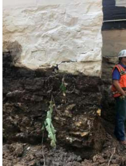
Excavation along the furnace room wall revealed that the wall did not reach the basement floor level or have a footing. This area will need to be underpinned with concrete to provide adequate support for the existing wall and to create an adequate base for the new addition.
